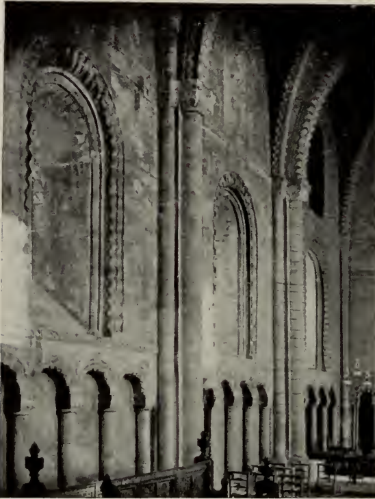
114. STOW, LINCS. ARCADE IN CHANCEL
